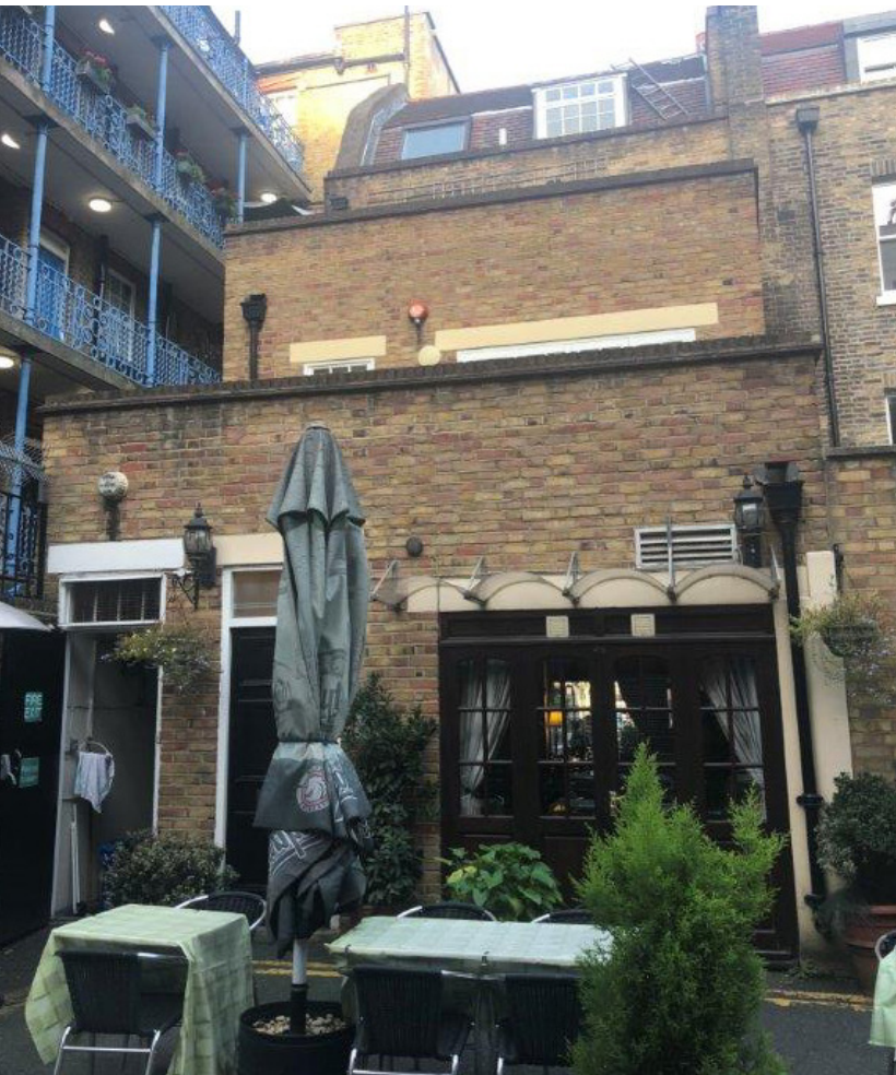
Rear of building (stedham Place)
